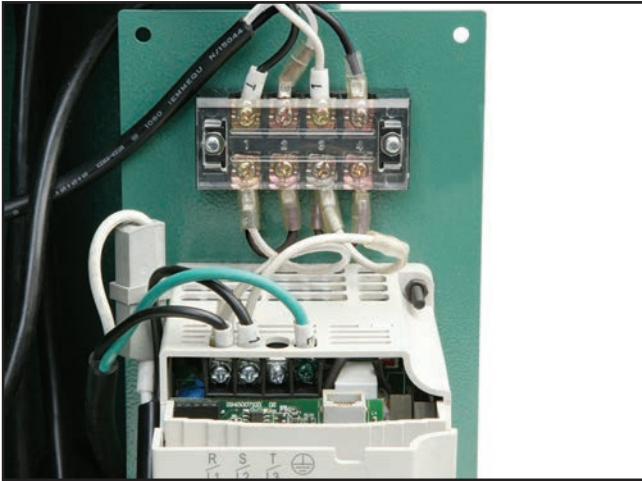
Figure 68. Upper half of power inverter.
